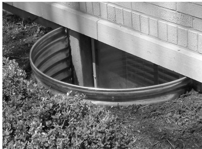
Standard window well installation
